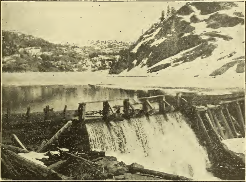
FIG. 4.—Spillway, Big Dam, South Fork Stanislaus River, Cal.
